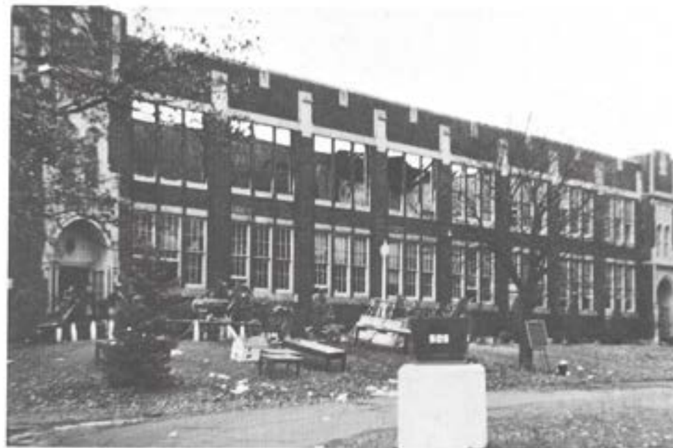
The School Building the morning after the fire of 1951.
