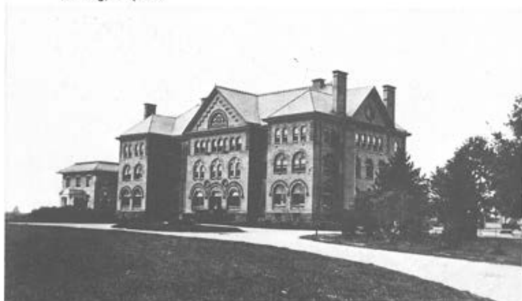
This is the oval in October 1911 with the new auditorium, adjacent to the Main Building, completed.
