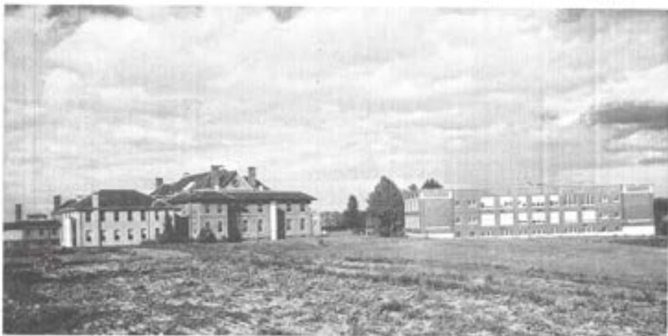
Back of School Building as seen from road.
