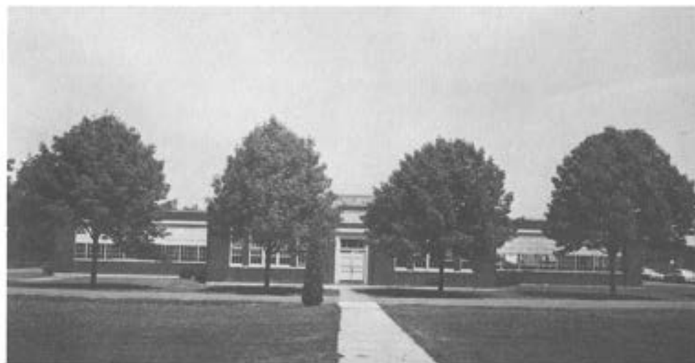
The Trades Building in 1955.
