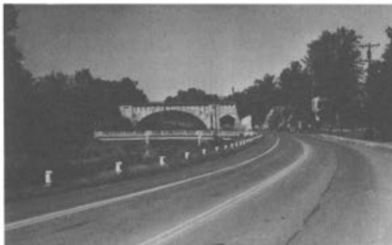
The same bridge was rebuilt of concrete in 1914. This is the way it looks from the other side today.
