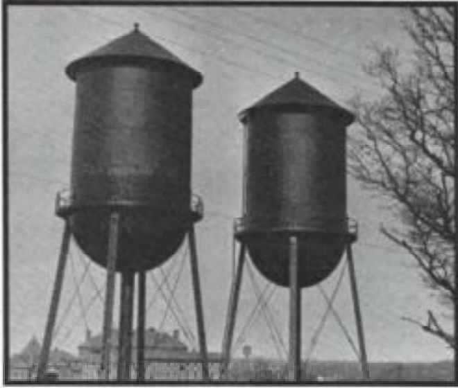
Above, left - The steel water tanks (100,000 gallons capacity each) erected on the southern edge of the campus along the Scotland-Chambersburg Road in 1914. They replaced the wooden tank which stood across from the lake in front of the farmhouse. Above, right- The Color Guard around 1919. In the center are the flag bearers Milbourn James (left) and Lester Cunningham. The Color Guards (outside) are unknown.
