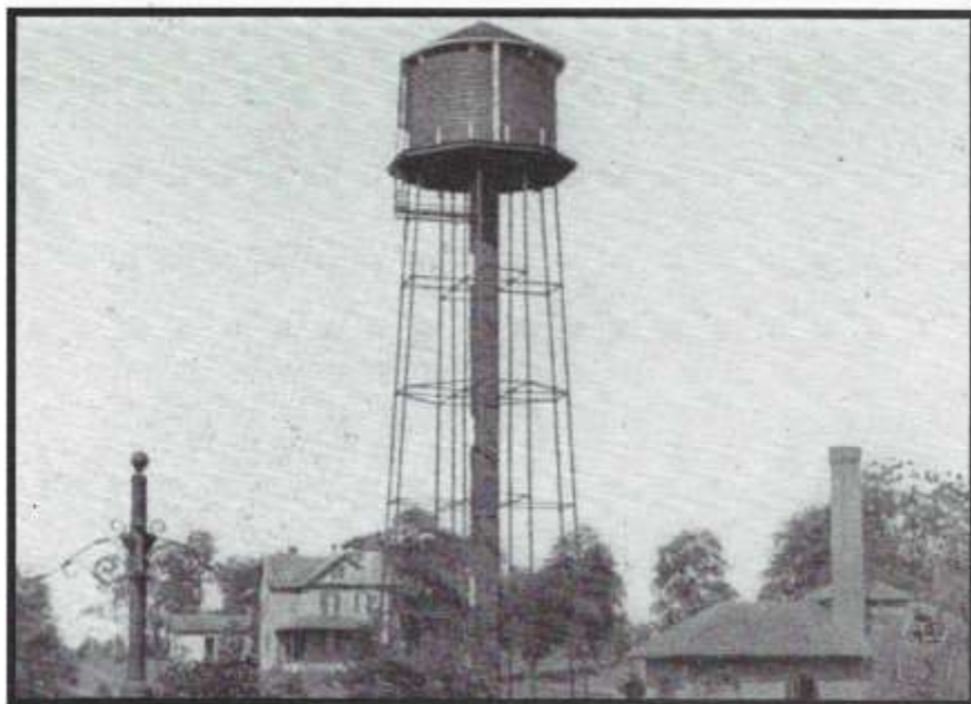
At the left is the 100,000 gallon water tank 30 feet in diameter and 20 feet high. It stood on a tower 110 feet high. Water came from four springs and was pumped to the buildings on the hill. Pump house is in the lower right.
